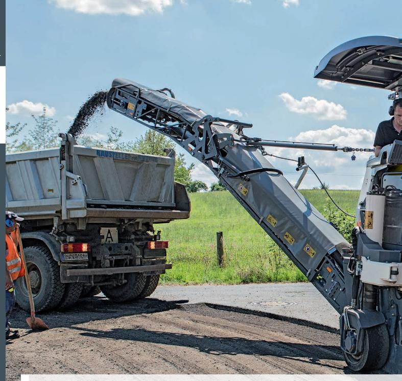
THE POWERFUL HALF-METER COLD MILLING MACHINE CONVINCES WITH ITS EFFICIENT OPERATING CONCEPT.
