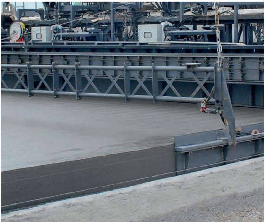
1-2 | Economical concrete paving at working widths ranging from 5.0 m to 16.0 m.
